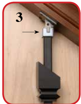
3 Snap Retaining Clip In Place
