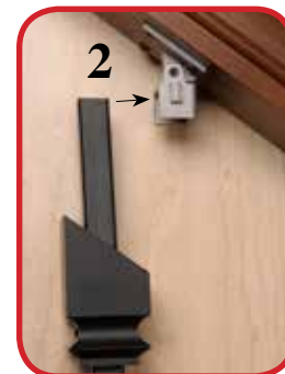
2 Slide Iron Baluster In Place With Shoes Installed
