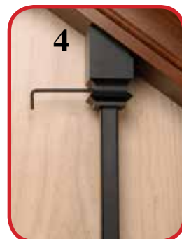
4 Slide Shoe In Place And Tighten
