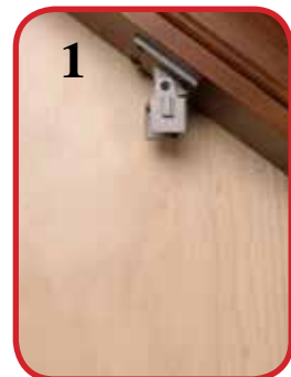
1 Install Clip To Handrail and Tread
