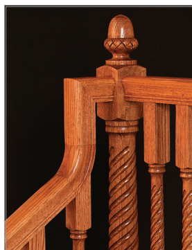
Cambered Post to Post
